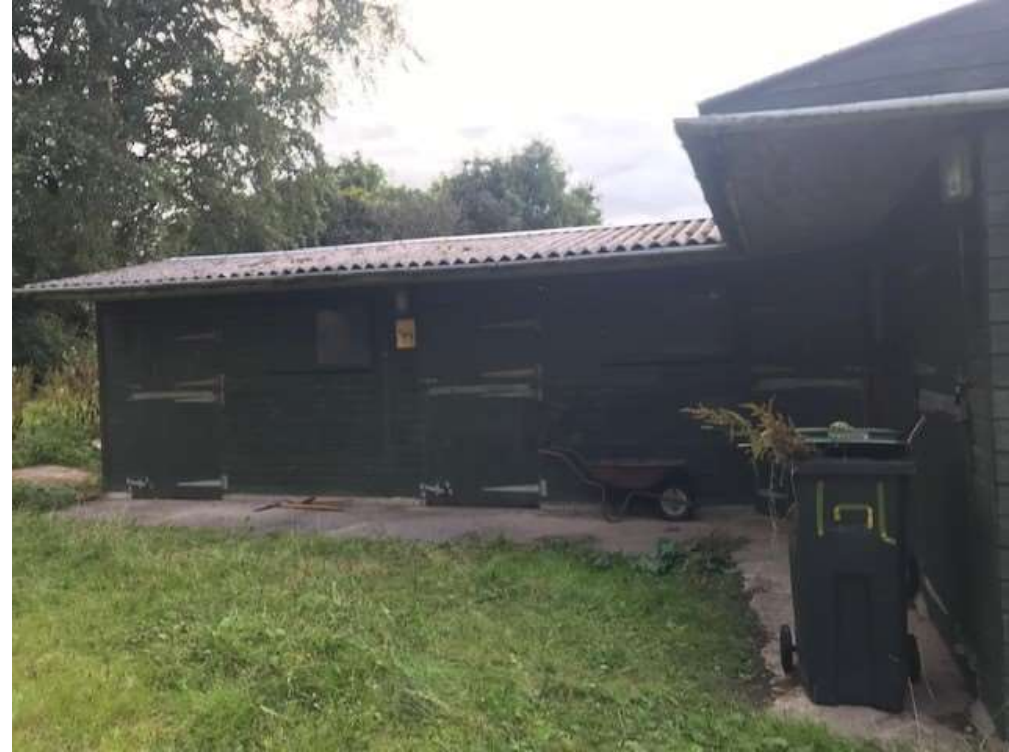
Figure 5. Eastern elevation of stables.
